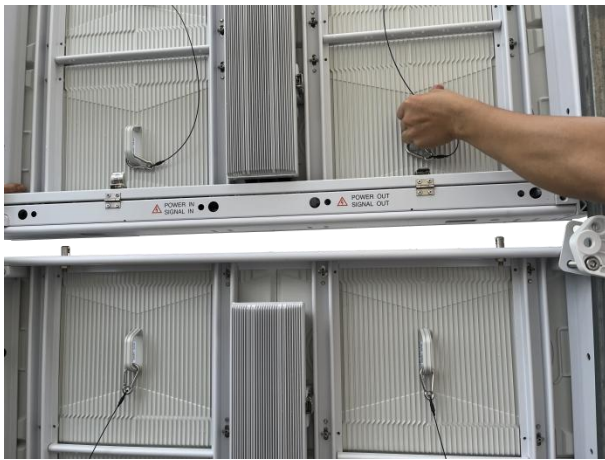
9) Put cabinet on top of the first row.
