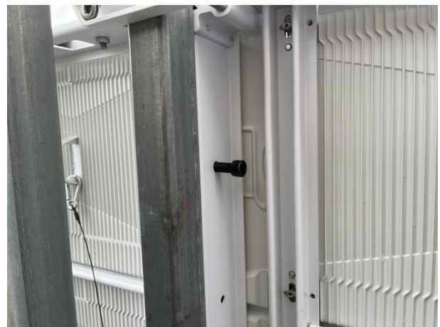
6) Put the screw through the cabinets.
