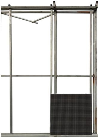
1) Prepare the structure and put the first cabinet.
