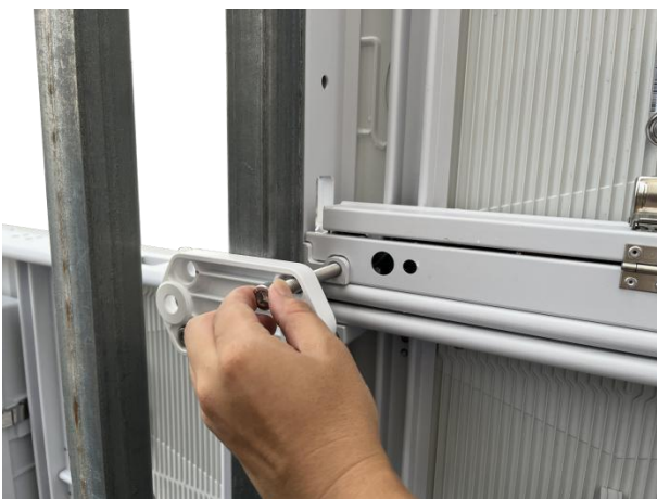
11) Put screws through the connection plate to the cabinet.
