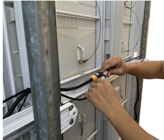
16) Connect cables together.
