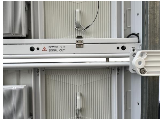
10) Locate the top cabinet with position pins.
