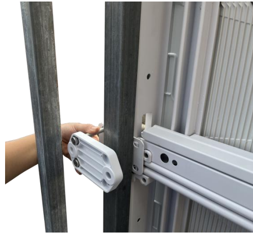
20) Put the connecting plates
