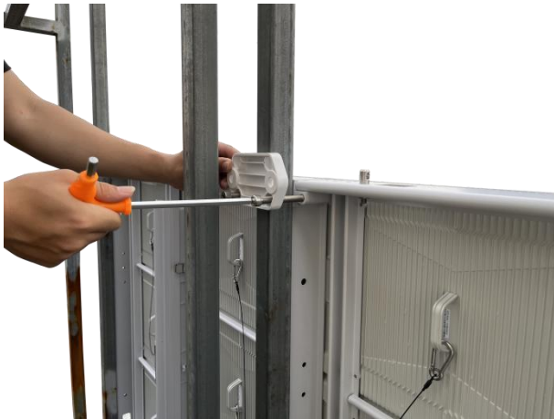
3) Lock the connecting plate to the cabinet with M10*75 screw from back.
