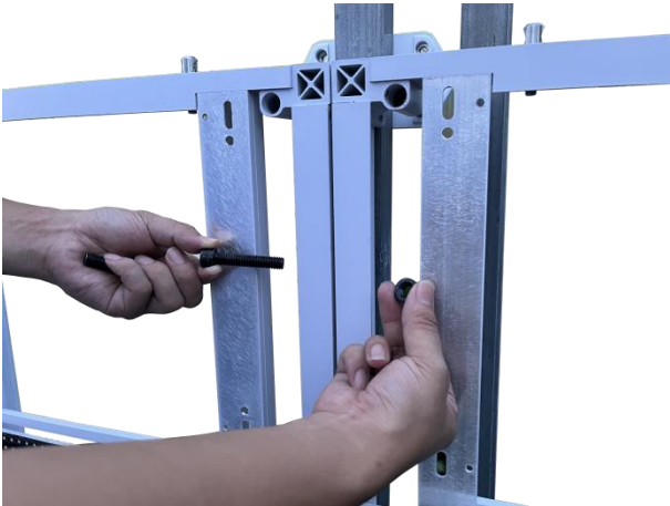
4) Connect two cabinets together with screws from side
