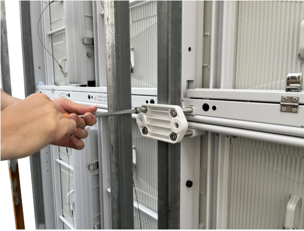
13) Fix all screws to the connecting plate
