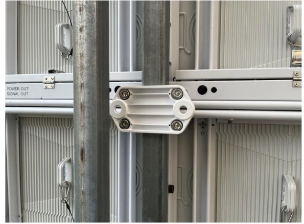
14) One connecting plate for 4 cabinets.
