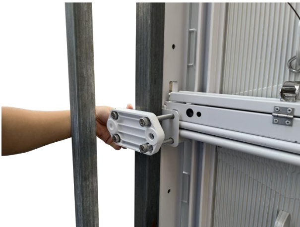
21) Lock the connecting plate with screws
