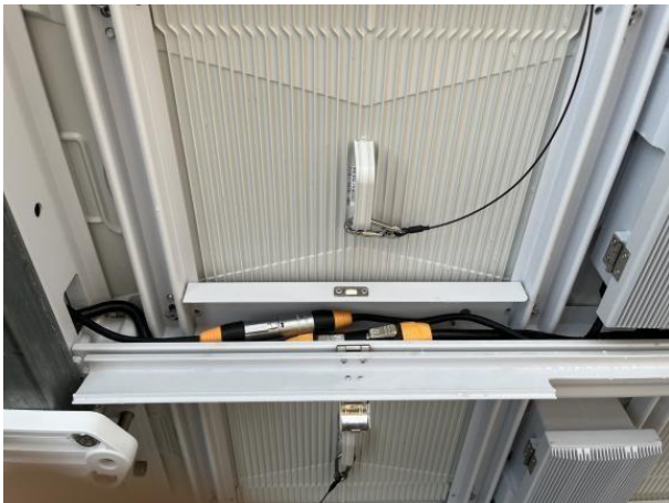
17) Put cables back to the cover.
