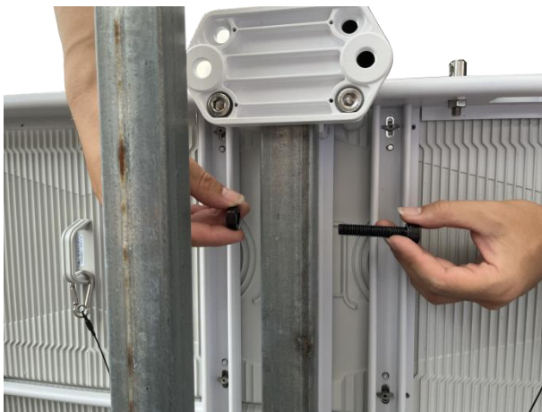
5) Connect left and right cabinets with screw and nut.
