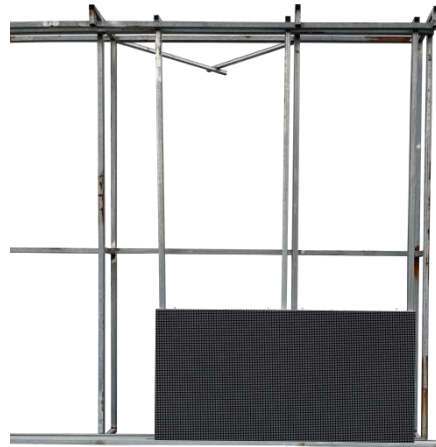
2) Put two cabinet together first.
