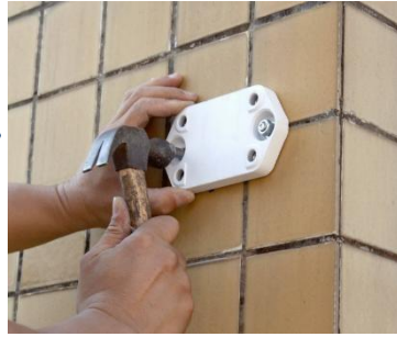
2)Locate plate with screw
