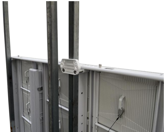
4) Lock two cabinets onto the steel square pipe.
