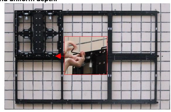
8. Align the mounting holes of the LDC500XX-LTP cabinet with the holes of the positioning slider and lock in with included M8 screws. Continue installing cabinets from top left, in a left to right and then top to bottom direction. Use the in built connecting locks to tightly join the cabinets together. Be careful to ensure that the cabinets are flat and uniform to each other.
