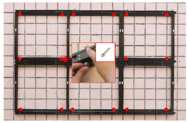
6. Join the next wall bracket in a horizontal direction and fix as per point 5, and then continue down, always working from top left, in a left to right and then top to bottom direction.
